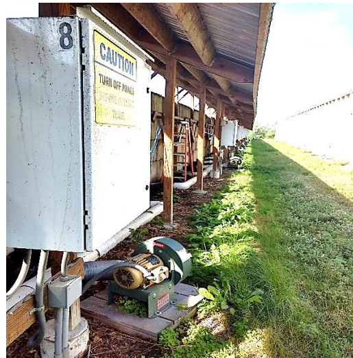
ASP Phase 2 ½ HP blowers
