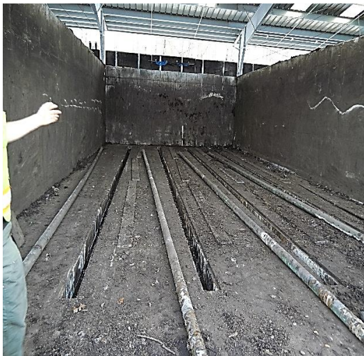
Phase 1 aeration trenches
