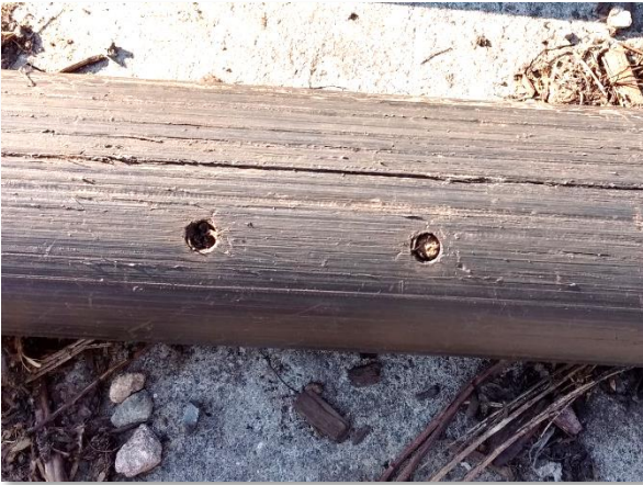
Clogged aeration hole
